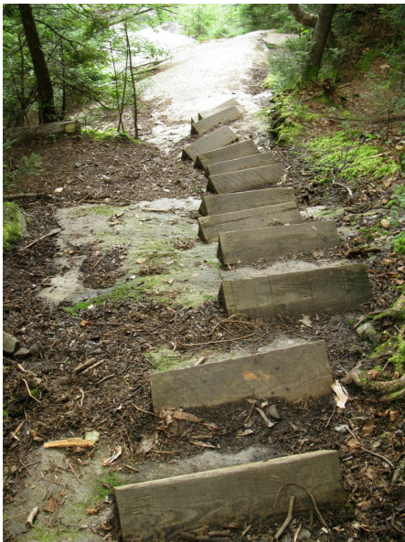
Wooden steps attached to the rock face
